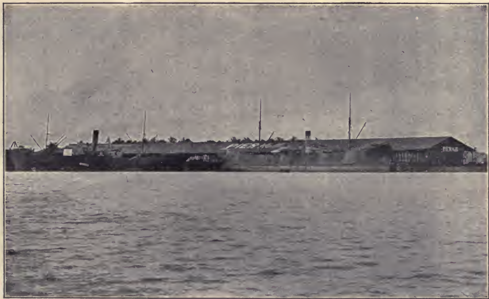
Pier 11 in the harbor of Cristobal.
